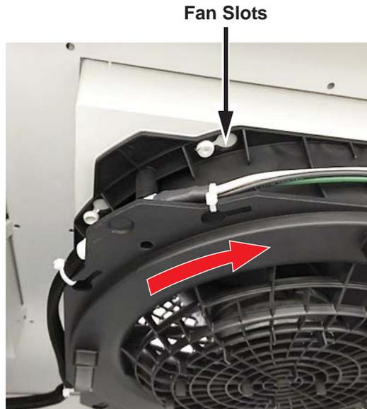
Figure 8: Fan back into position after filter removal.
