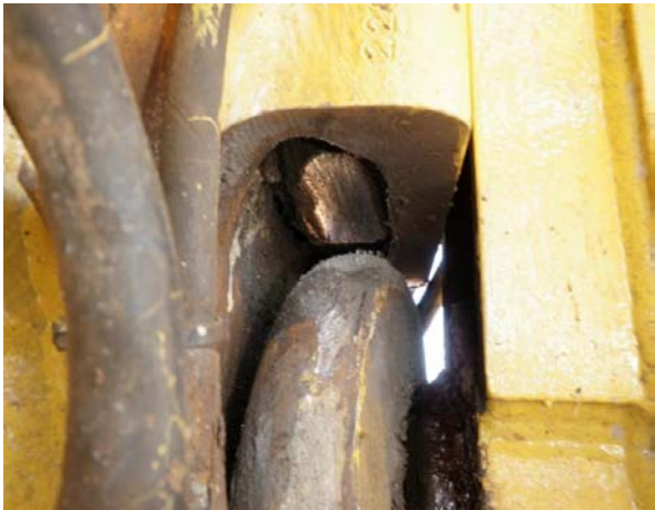
Figure 2: Wear evident on split block adapter as a result of continuous contact with elevator link
