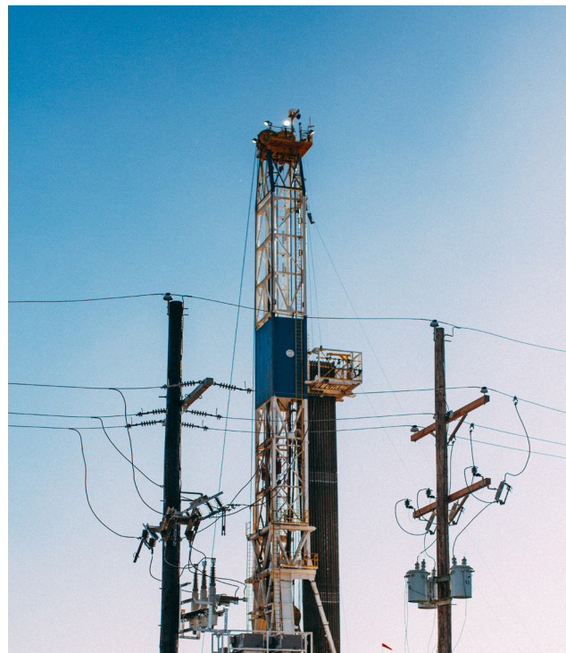
Rig electrification using high-line power offers a lower carbon alternative to diesel engines.
