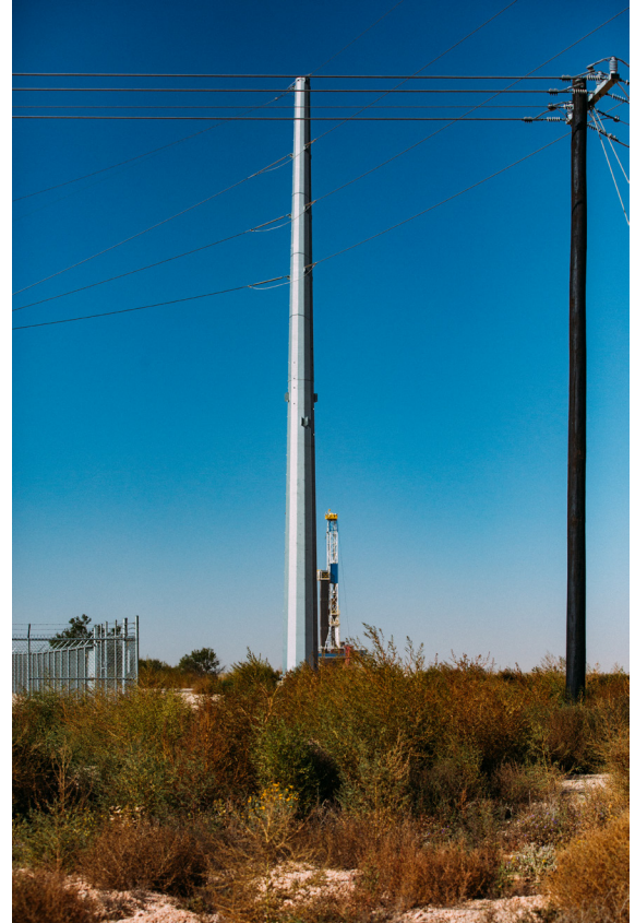
Photo: PACE®-X Rig in Texas
